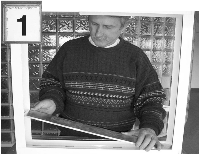
Place sill infill in bottom of frame.
