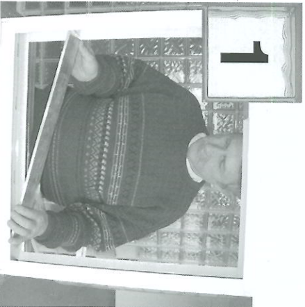
1 Place sill infill in bottom of frame.
