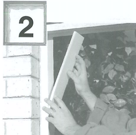
2 Place the Ezylay expansion material in both verticals of the Ezylay frame ensuring it extends from top to bottom.
