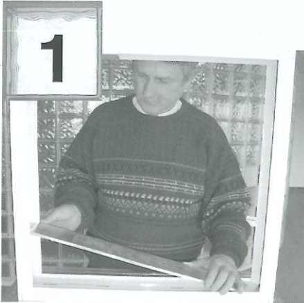
1 Place sill infill in bottom of frame.
