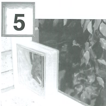
5 Place the first row of glass blocks in the frame sill, supporting and spacing each block with a "T" connector.
